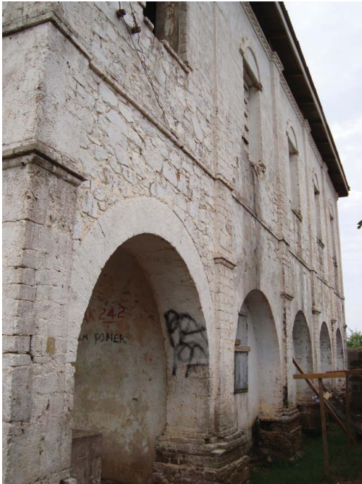
Figure 1. Amonoo Residence, South Façade, Kwamin Atta Amonoo, 1920, stone nog, brick, concrete (paint added later), Anomabo, Ghana. 2009 (author’s photo).
