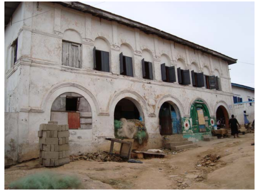
Figure 13. Allen Quansah Family Residence, c. 1883, stone nog, brick (cement plaster and paint added later), Cape Coast, Ghana. 2009 (author's photo).
