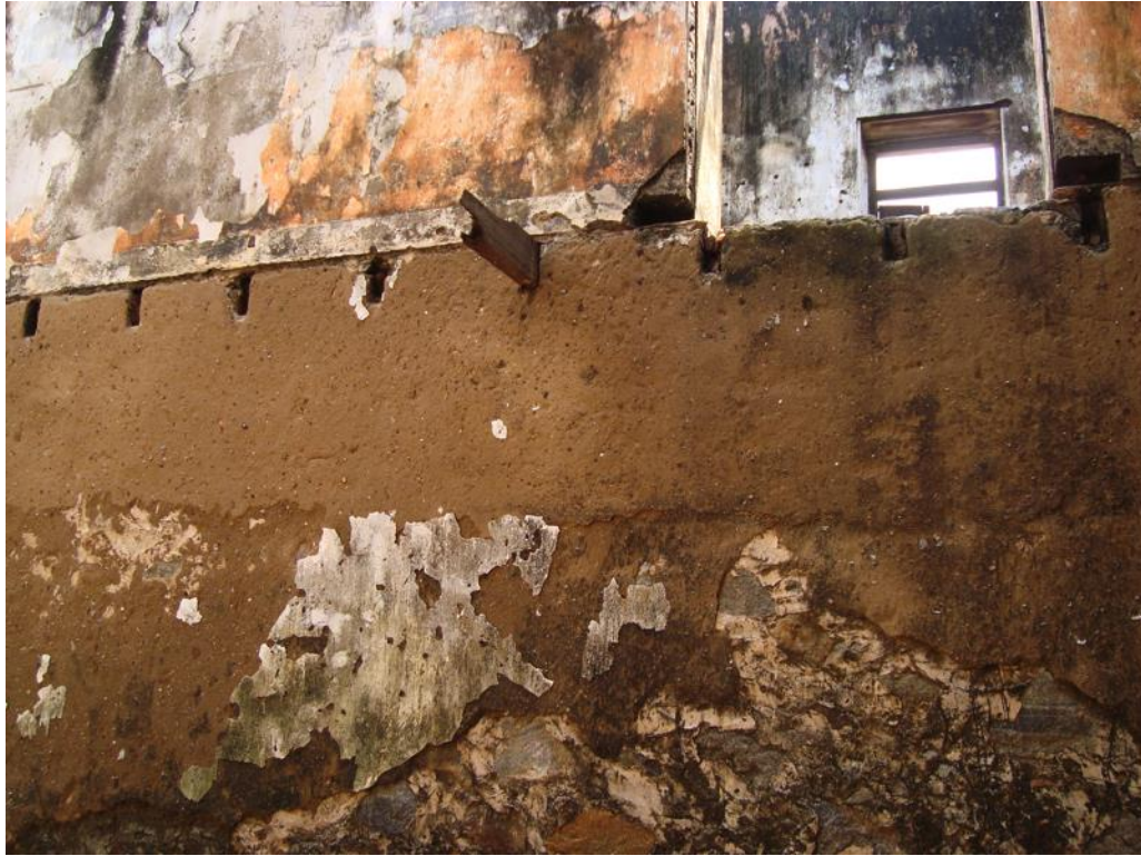
Figure 12. Russell House, plaster walls. 2009 (author's photo).
