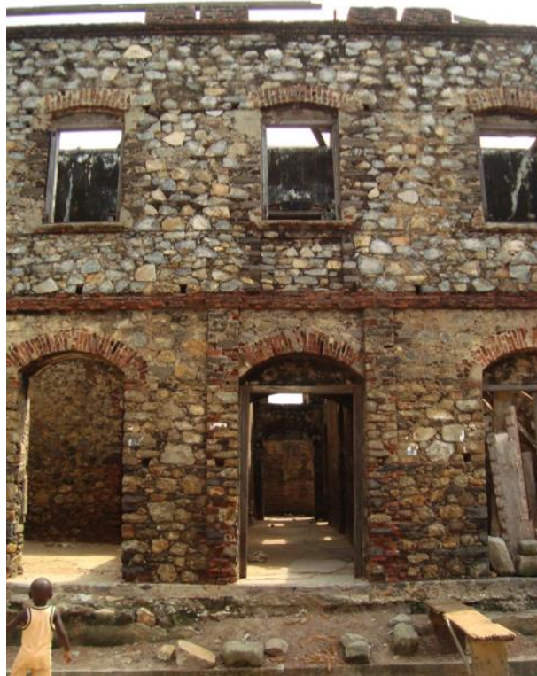
Figure 13. Russell House, entrance. 2009 (author's photo).
