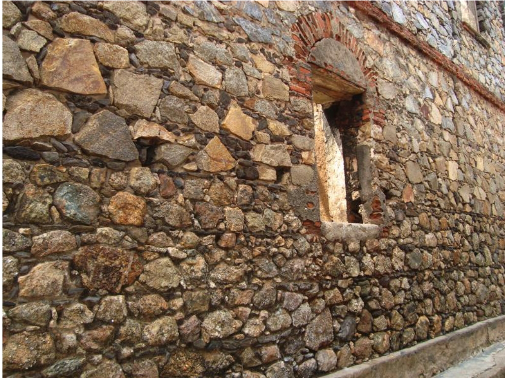
Figure 10. Russell House, wall surface. 2009 (author's photo).
