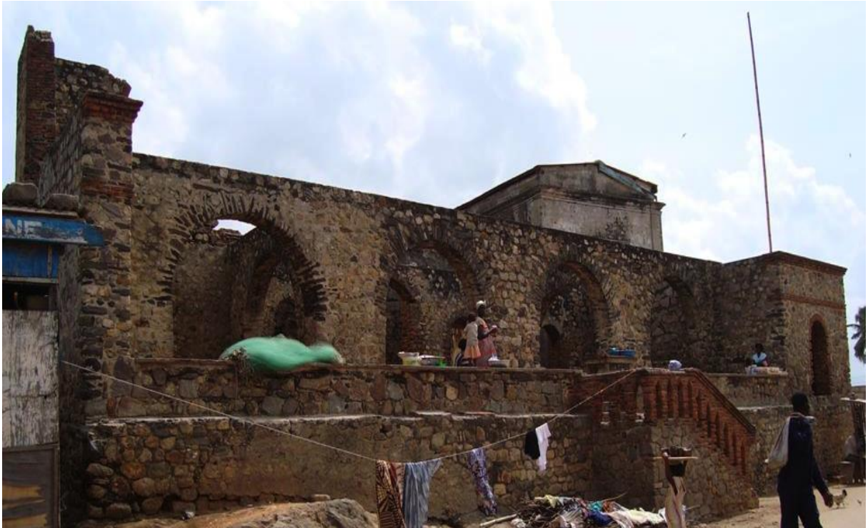
Figure 8. George Kuntu Blankson Addition, South Façade, Castle Brew, c. early 1870s, stone nog, brick, Anomabo, Ghana. 2009 (author's photo).
