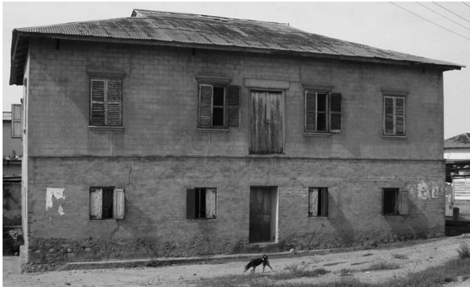
Figure 9 Justice Akwa family residence, ca. 1900, stone nog with brick facing (cement plaster on the second story added later), Anomabo, Ghana, 2008 (author's photo).
