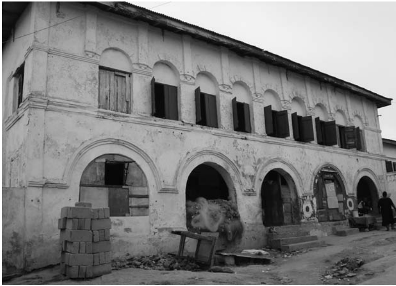
Figure 24 Allen Quansah family residence, ca. 1883, stone nog , brick (cement plaster and paint added later), Cape Coast, Ghana, 2009 (author's photo).
