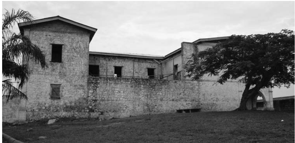
Figure 20 Amonoo family residence, west side, Kwamin Atta Amonoo 1920, stone nog , brick, concrete (paint added later), Anomabo, Ghana, 2009 (author's photo).
