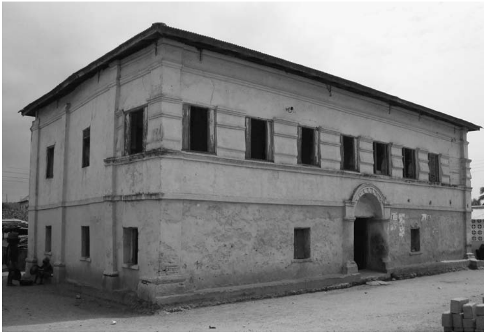
Figure 14 Kobena Mefful family residence, ca. 1900, stone nog with brick facing (cement plaster and paint added later), Anomabo, Ghana, 2009 (author's photo).
