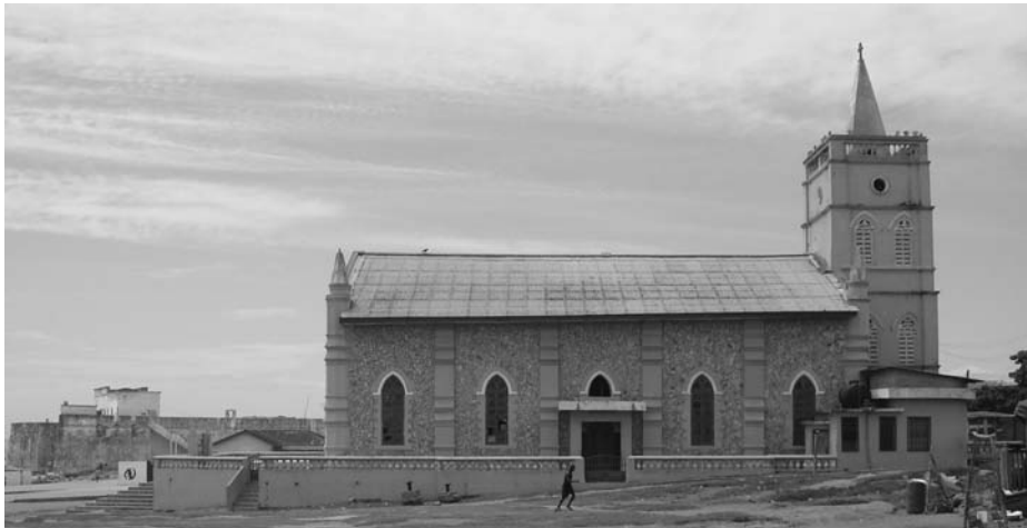
Figure 19 Ebenezer Methodist Church, Revs. James Picot, James Fletcher, and John Oboboam Hammond, 1895, stone nog . Renovation 1966–71, rebuilt main entrance façade, stone nog , cement, and paint. Anomabo, Ghana, 2009 (author's photo).
