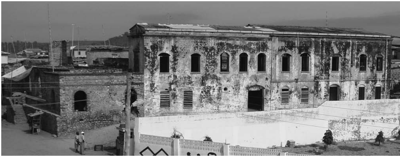
Figure 4 The Castle Brew compound includes the original Castle Brew, far right; the Cruickshank Addition, middle; and the Blankson Addition, unplastered on left. Original Castle Brew, Richard Brew, Irish, ca. 1761–63; Cruickshank Addition, Brodie G. Cruickshank, Scottish, ca. 1841–44; Blankson Addition, George Kuntu Blankson, Fante, ca. late 1860s–early 1870s. Stone nog , brick (cement plaster and paint, added in the 1960s to the original Castle Brew and Cruickshank Addition), Anomabo, Ghana, 2009 (author’s photo).
