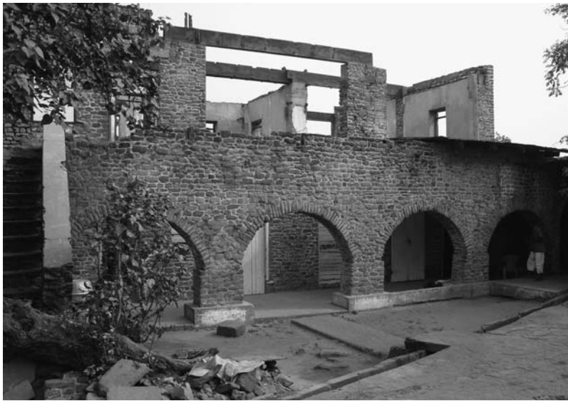
Figure 8 Franklin House, Danish patron(s), ca. 1800, stone nog , brick, Jamestown, Accra, Ghana, 2012 (author's photo).
