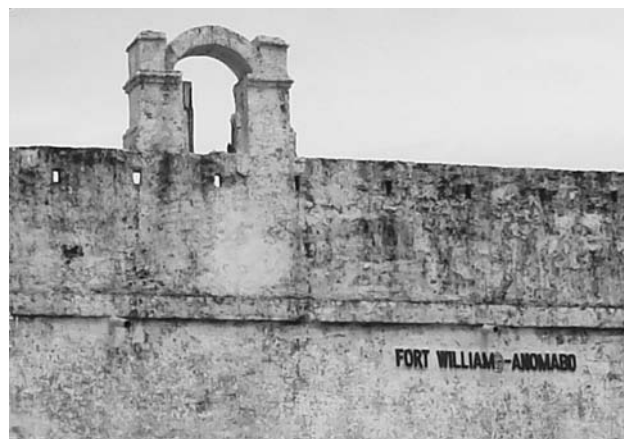
Figure 16 Fort William, north side, 1760 and 1840s, stone nog (paint added later), Anomabo, Ghana, 2008 (author's photo).
