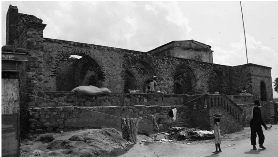
Figure 6 George Kuntu Blankson Addition, South Façade, Castle Brew, ca. late 1860s to early 1870s, stone nog , brick, Anomabo, Ghana, 2009 (author's photo).
